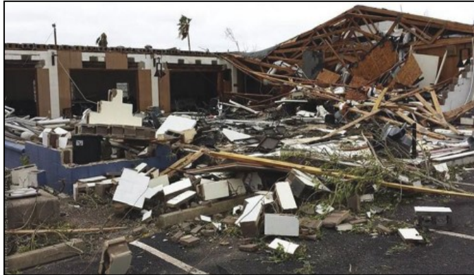
Remains of VFW Post 3904 in Rockport, Texas after Hurricane Harvey passed through the area.
